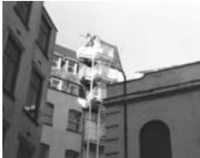
Clements Lane fire escape
